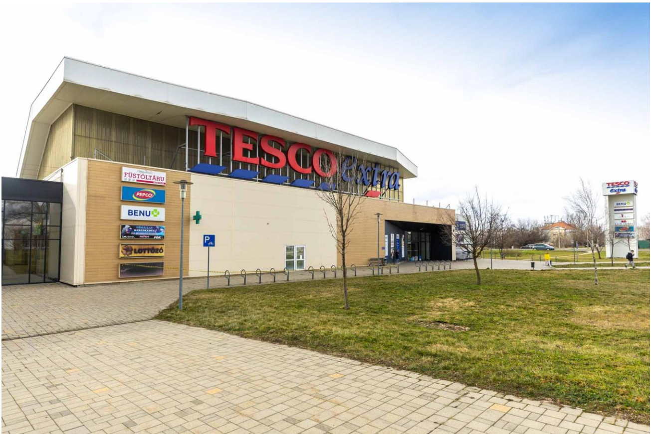
1. Figure Picture of of the building
